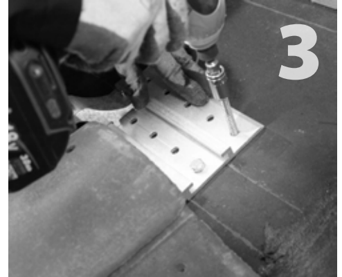
3 Connect hook (item 3) to base plate and drive lag screws (item 2) into rafter through the two holes to a solid, snug fit. DO NOT over tighten lag screws, this may compromise their holding strength.
